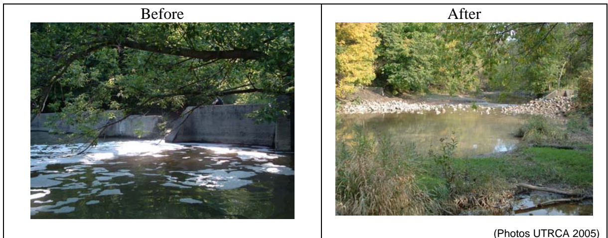
Figure 2.2: Dingman Weir Before and After
