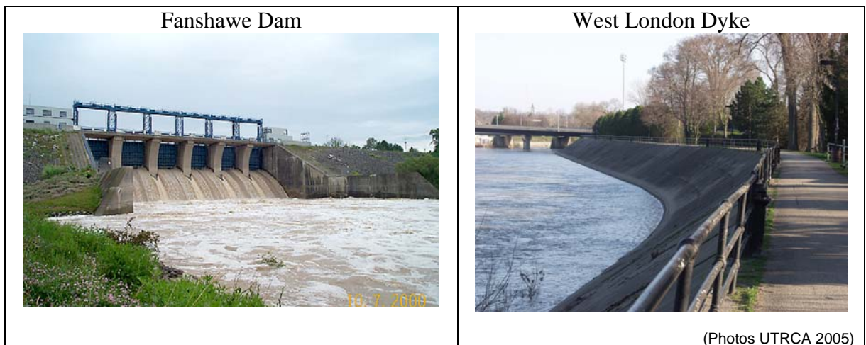
Figure 2.1: Examples of Flood Control Structures in the Upper Thames River Watershed
