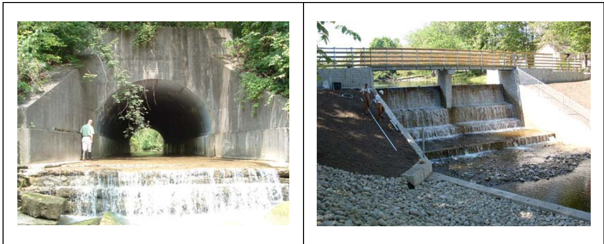
Figure 4.9: Oxbow Creek Rail Culvert and Dorchester Mill Pond Dam
